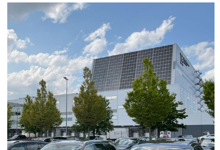
Abb. 26 Fassaden-Photovoltaik, Hochregallager Heinemann in Erlensee
