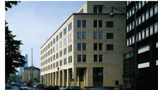
DZ-Bank Büroturm / DZ-Bank office tower Frankfurt am Main Generalplanung / general planning 1999-2002
